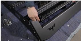
4. Next we will install the mounts to the rack. The mounts will have letters cut out on them to determine if they are front (F) or rear (R) mounts. The letter side of the mounts will attach to the roof of the truck. Make sure the arrow is facing toward the front fairing before bolting it on. Use 2 button head bolts with washers and flange nuts then secure the mounts on the inside of the rack. The access cab will only have front and rear mounts.
