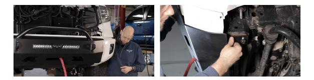
**11.** Using a 14mm wrench, adjust the height of the bumper wing (with the bracket we installed earlier to the light bracket).
